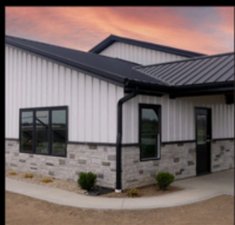
STEEL ROOFING & SIDING
